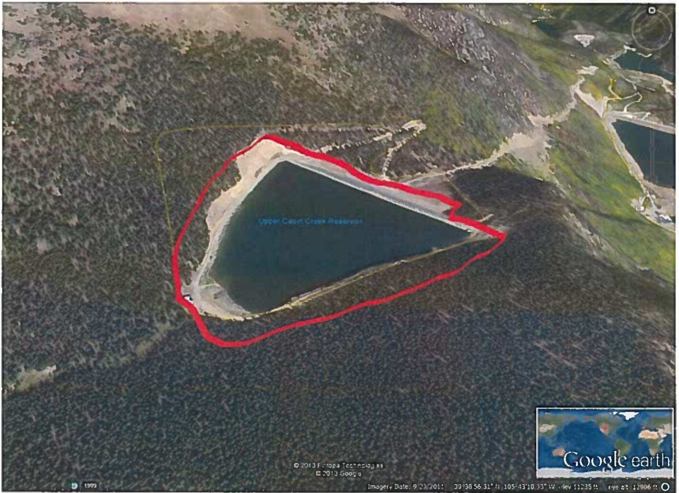
Figure xx: Upper Cabin Creek Reservoir
